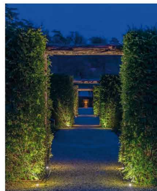
Figure 73: Uplight from ground to colonnade archway
