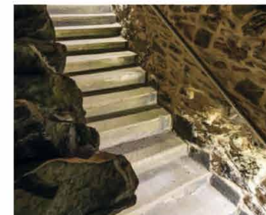
Figure 70: Light within handrail to steps
