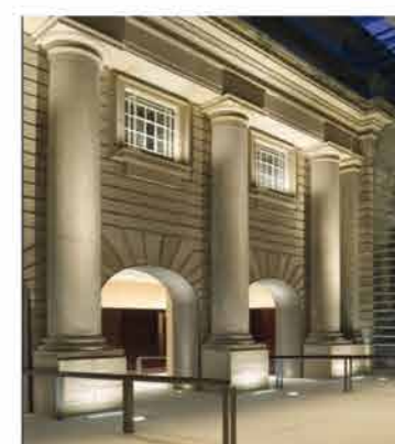
Figure 53: Main facade uplit from ground recessed luminaires
